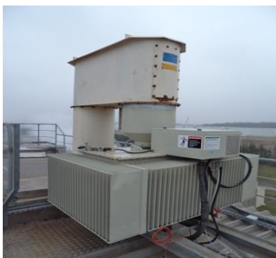
Fig 1: Three phase TR at Luxemburg
