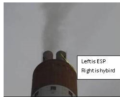
Figure 11 Emission comparison of ESP and ESP-FF hybrid dust collector
